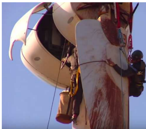
Figure 1. Manual cleaning of wind turbine blades.
