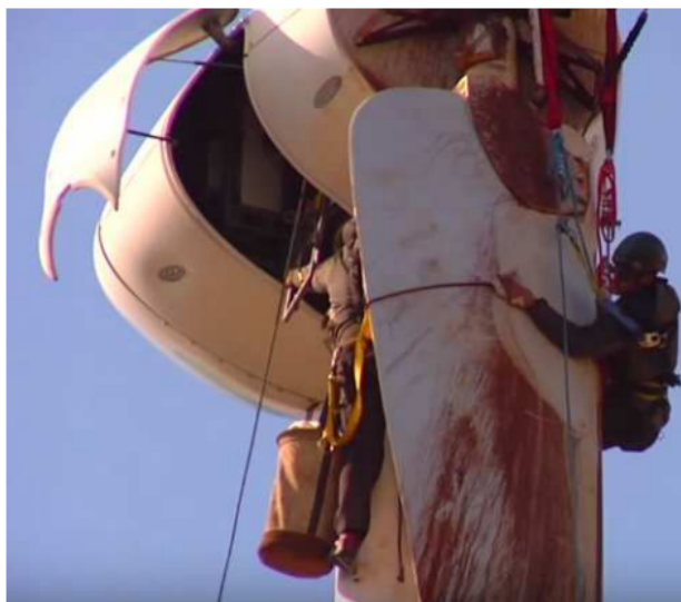
Figure 1. Manual cleaning of wind turbine blades.
